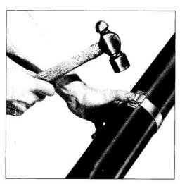
Clinch stub by hammering down buckle ears, completing the clamp.
